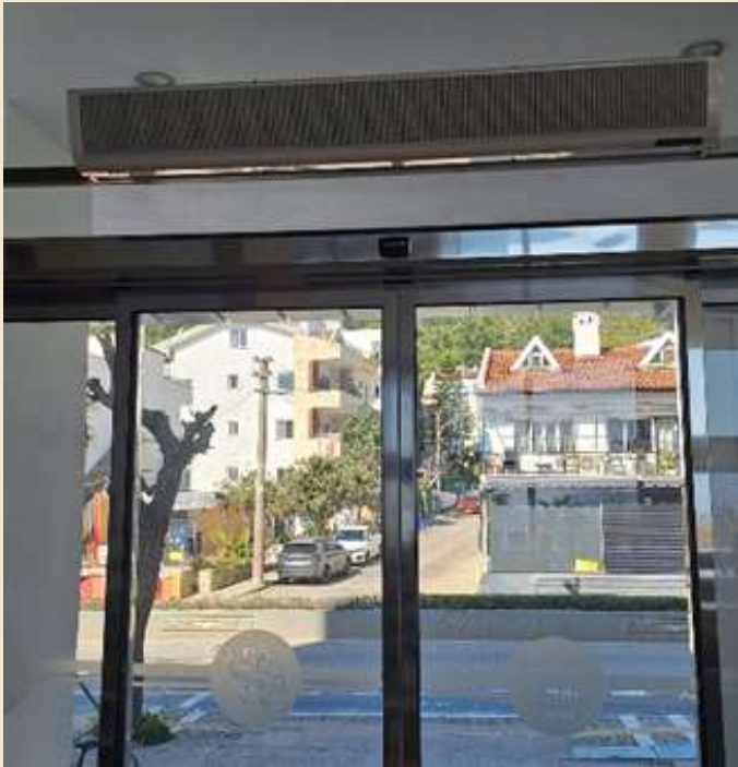
Environmentally friendly external door air curtain
